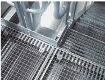
Fig. 35: Toe-plate on the substructure
